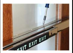
6) Attach the Top Cover with supplied screws to capture the shims and secure the Shim Kit Assembly
