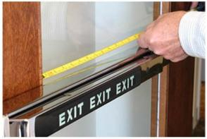
Measure door's recessed area. Cut Top & Bottom Covers to match/ accommodate the contour of the recessed area or the shape of the window frame
