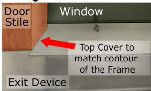
Cut the Black Nylon Back Plate and Shims to fit under the rail assembly; Match the contoured ends to the recessed area or the window frame. Remove all burrs
