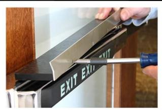
Attach finished Bottom Cover to Black Nylon Back Plate with supplied screws
