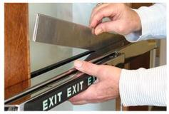
5) Insert supplied shims to fill the gap between the backside of the rail and the Black Nylon Back Plate
