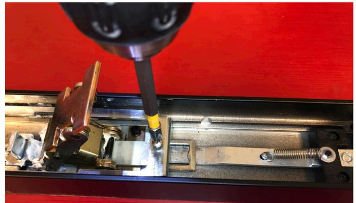
7. Behind plunger bracket, install solenoid mount by sliding one side into the middle groove.
