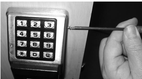
FIG. 17: SECURE THE TOP OF THE SECONDARY HOUSING
