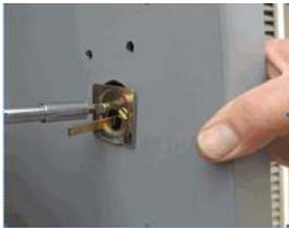
1. Using the supplied template, drill the appropriate hole in the door in order to mount a CER-KD rim cylinder.
