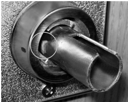
FIG. 6: PUSH IN LEVER CATCH
