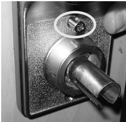
FIG. 16: SECURE THE SECONDARY TO THE PRIMARY HOUSING
