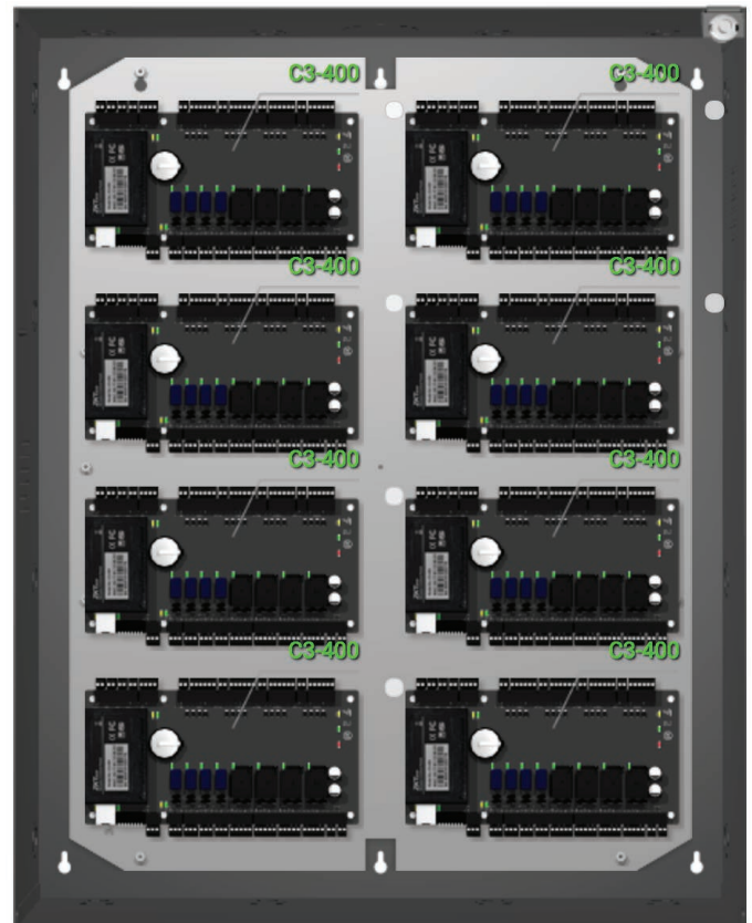
32-Door Access System
