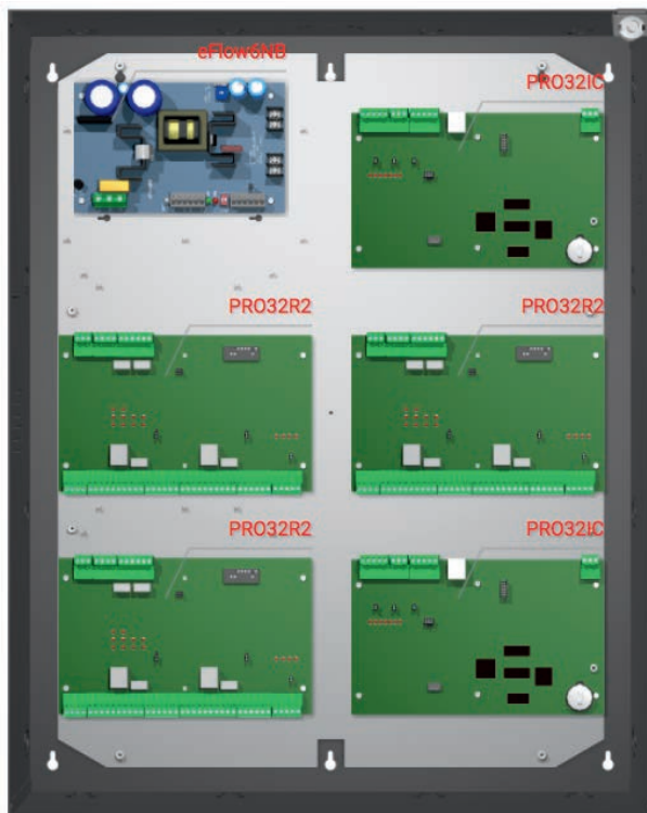
10-Door Access System (ProWatch) with Power
