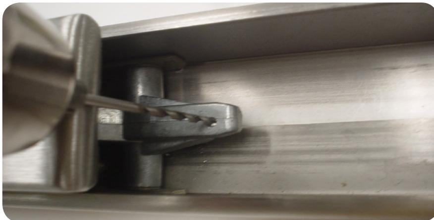
E. Test Rex switch for proper operation and adjust if necessary
