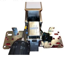
$6. \ \, \mbox{PUSH THE TWO TABS ON THE LBM BRAKET INTO THE EXISTING HOLES IN THE EXIT DEVICE HEAD.}$
