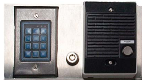
Install a keypad & intercom.
