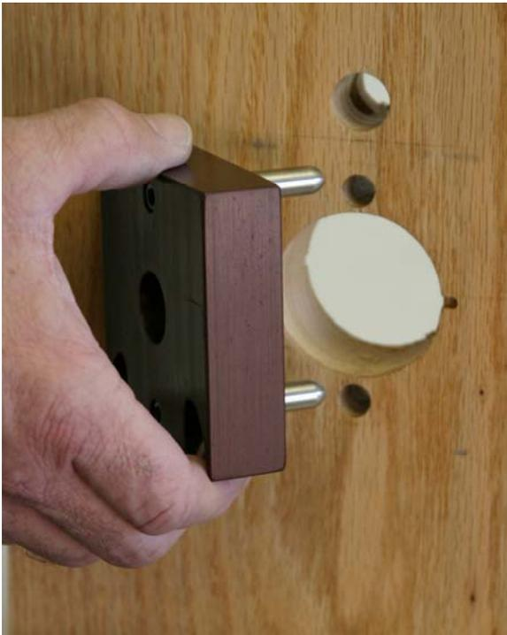
Install the wire run guide over the cross bore using the two alignment pins. Bolt to the backplate with the 3/8" allen bolt. Mount this guide on the battery side of the door.
