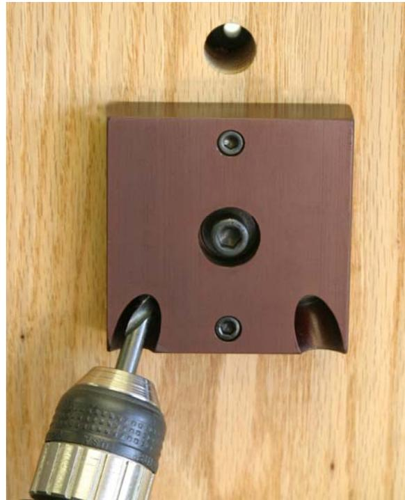
Drill for the wire run using a 5/16" drill bit. Choose the bushing that will allow you to drill from the hinge side of the door to the latch side of the door.
