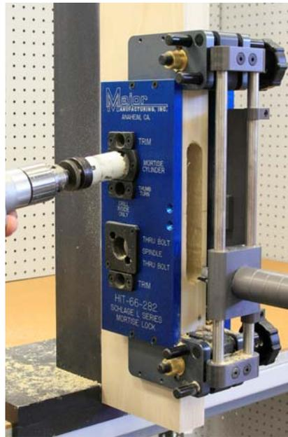
Mortise cylinder hole being drilled to the pocket on the outside of the door.
