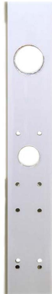
Here is the completed door prep. Make sure all holes have been de-burred and install lock per manufactures directions.
