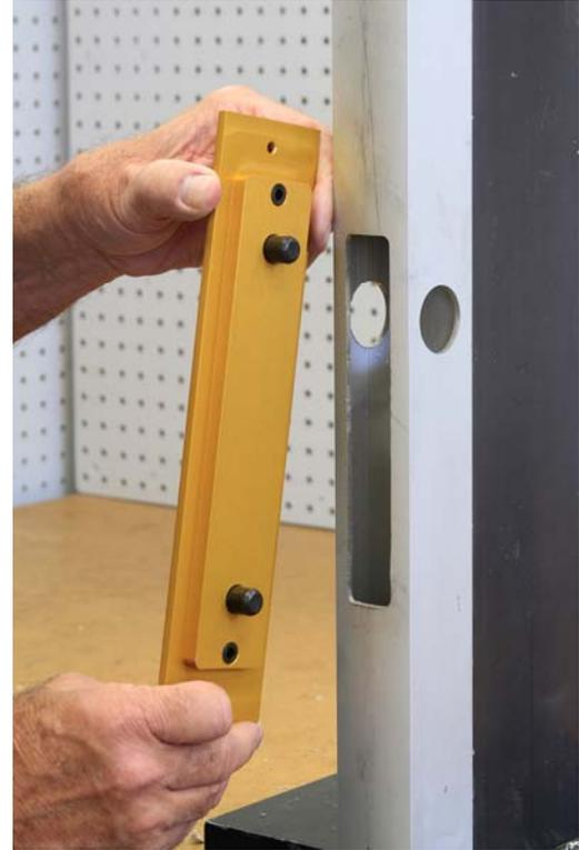
If this installation is new, a faceplate will need to be cut in the door, attach a HIT-30AR11 to the clamp. (LH picture) If you are retrofitting an existing door prep, attach a HIT-30AR20 alignment guide to the clamp. (RH picture)
