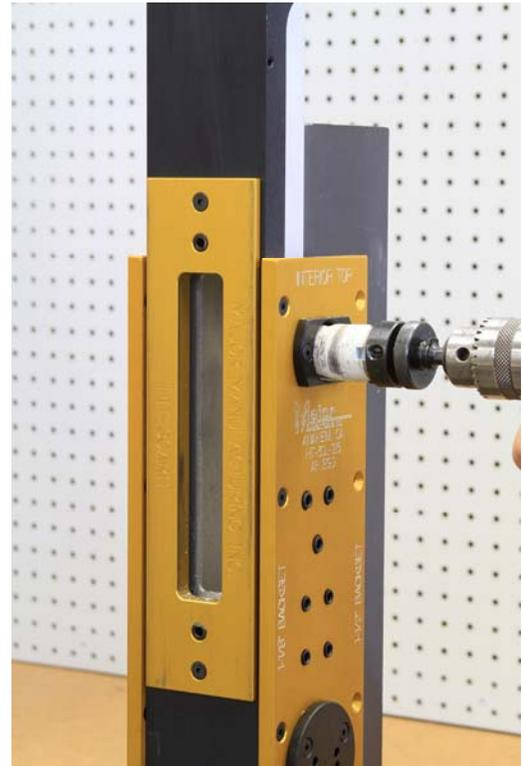
Once the faceplate has been cut out it is time to start drilling the function holes. Starting at the top, drill the inside and outside holes with a 1-1/4" hole saw. If retrofitting, drill these holes to clean up any misalignment.
