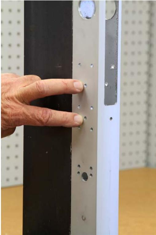
On the exterior template two holes need to be enlarged to 1-1/8" with the use of a hole saw. One hole is located in the center of the door, below the two horizontal holes. The second hole is centered between the bottom five holes.
