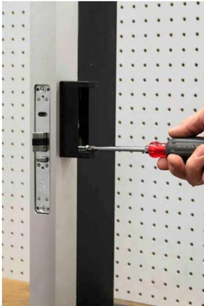
Install paddle handle with fasteners top and bottom. Add push paddle with hinge pin and finally lock face plate.
