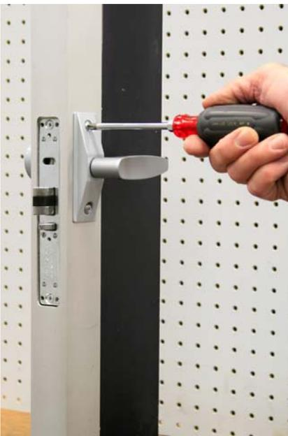
Install mounting screws both top and bottom and install the lock faceplate.
