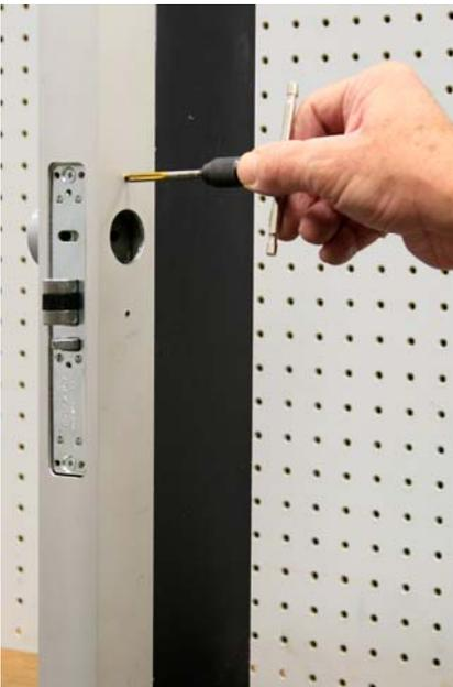
Remove drill guide and tap both holes with a 10-32 tap.
