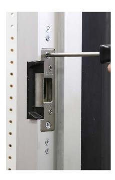
Install strike to factory mounting tabs and tighten all of the mounting screws.
