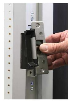
Connect the wire leads and insert strike into the frame.
