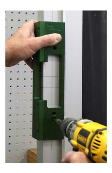
Align the HIT-41 template to the pencil marks and attach to the jamb using tek point dry wall screws. It is a good idea to use a drill with a clutch feature, you don't want to snap the screw off in the jamb.
