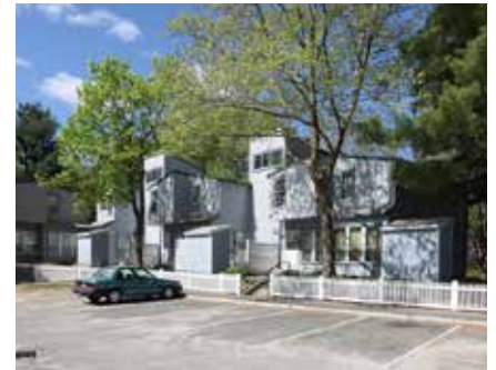
SPRINGFIELD APARTMENTS Springfield, MA
