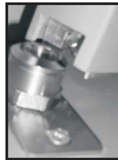
Figure 2b: Door placed on top of 218 Pivot.
