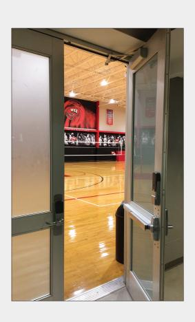
team's time, they can also create safety and security risks on campus. If the rods aren't performing correctly, they can keep the door from latching, like the case in Diddle Arena. If not corrected, unlatched doors can cause security issues.
